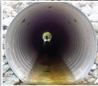
2800 mm diameter corrugated steel pipe liner in place showing capped grout fittings.
