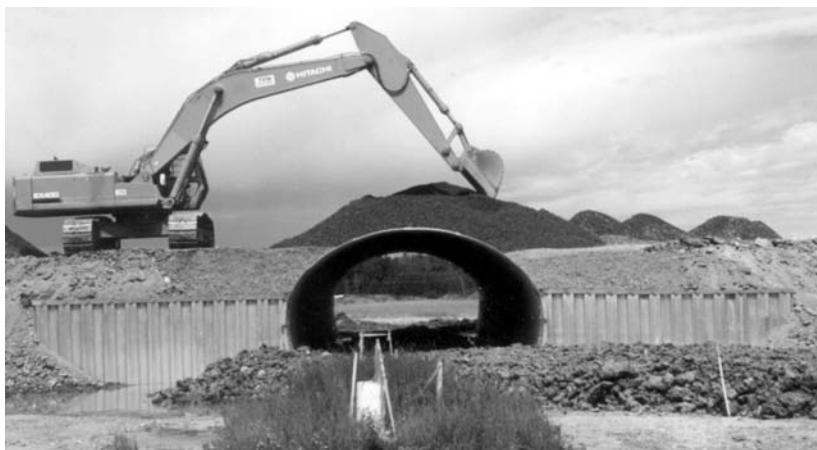
Cold-formed sheet steel piling prevents erosion.
