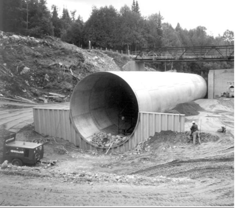
Cold-formed steel sheet piling serves as end wall for CSP.
