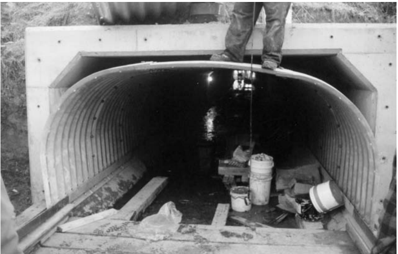
Lining a concrete box with a steel box culvert.
