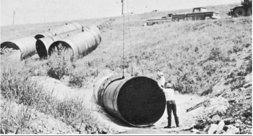
Sliplining a concrete culvert with steel pipe.
