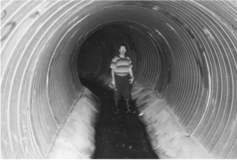
Concrete paved invert.
