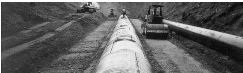
Compaction parallel to pipe.
