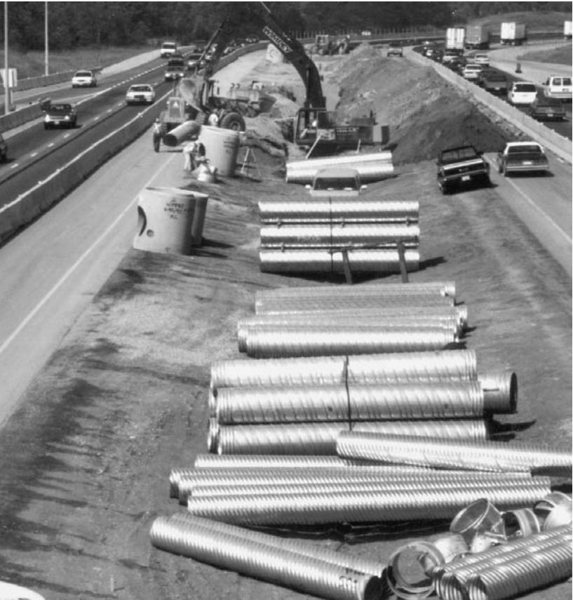
Traditional CSP and Spiral Rib Pipe on highway 401 near Toronto, Ontario.
