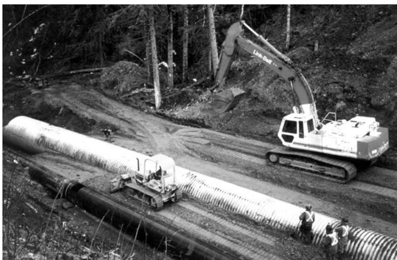
CSP installation with straight alignment.
