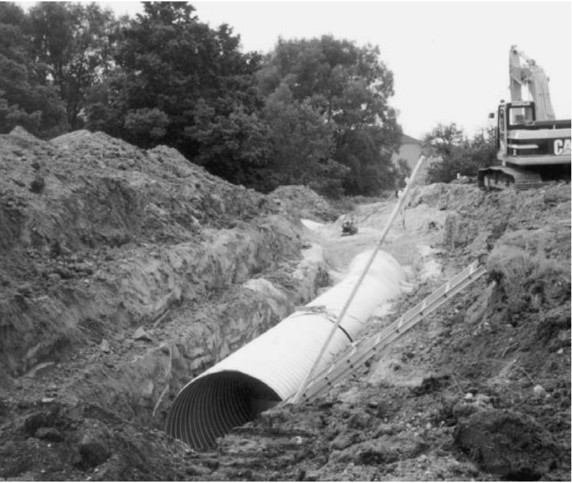
Spiral rib steel pipe stream diversion installation.
