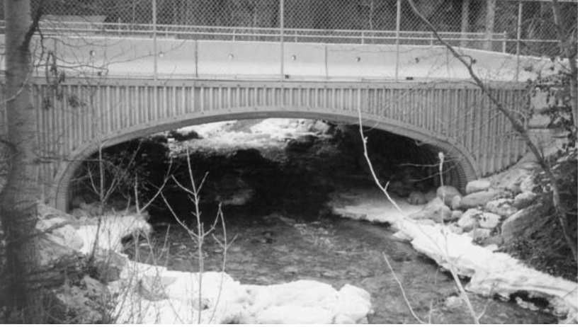
DCSP box for a short span bridge.
