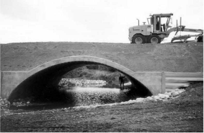
Low profile arch with concrete and bin-type retaining wall end treatment.
