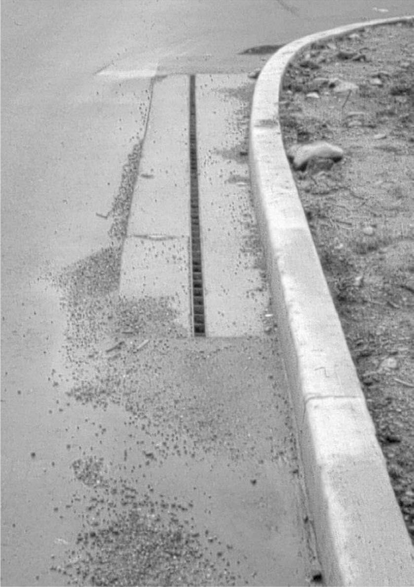
CSP slotted drain inlet.
