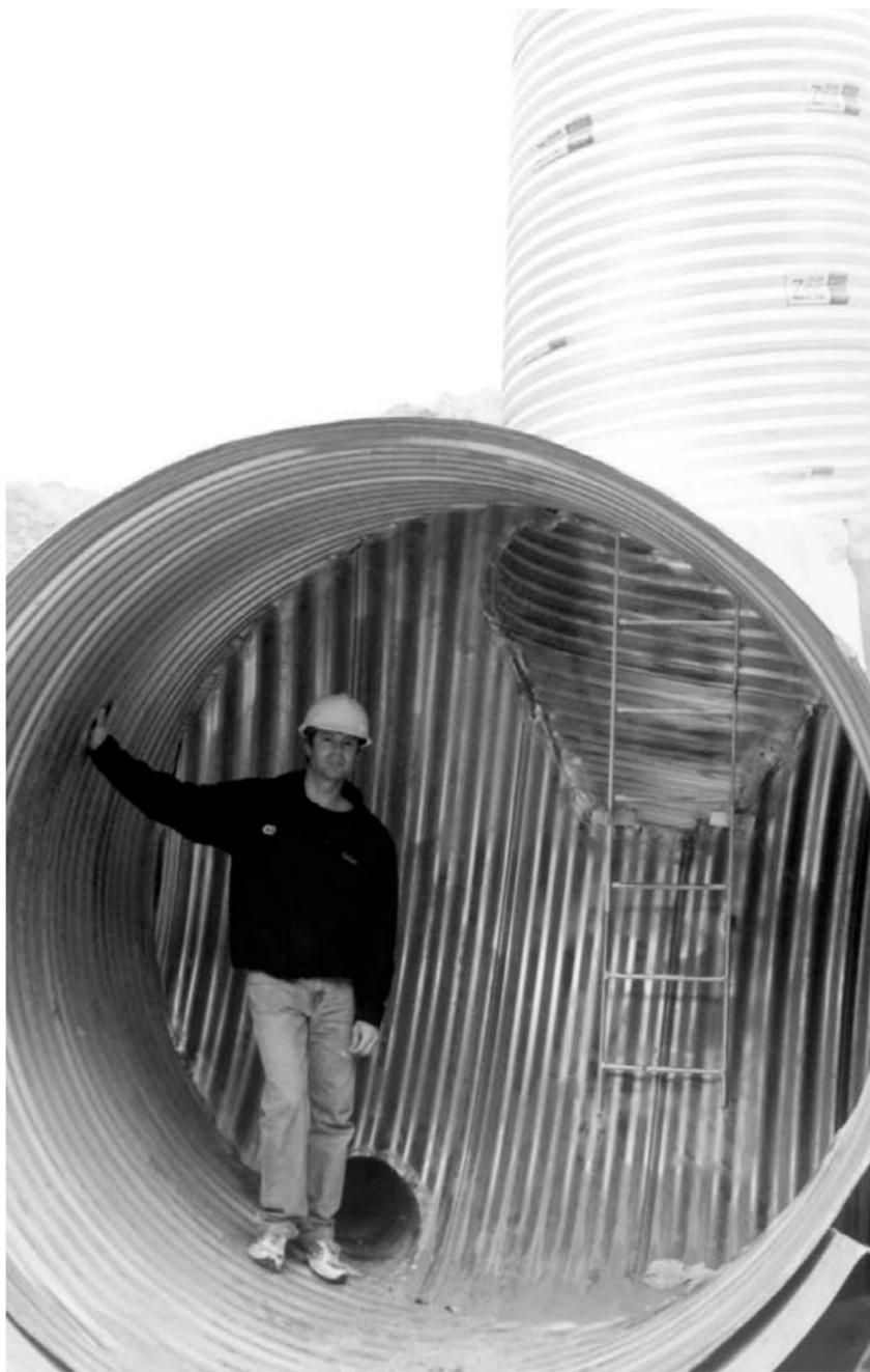
Fabricated riser type CSP manhole.
