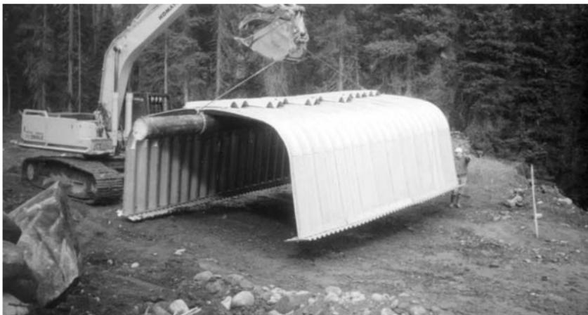
Deep corrugated structural plate box culvert assembled at job site.
