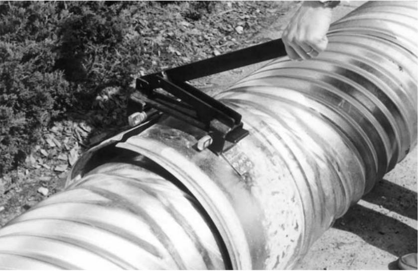
A band puller eases installation of coupler.
