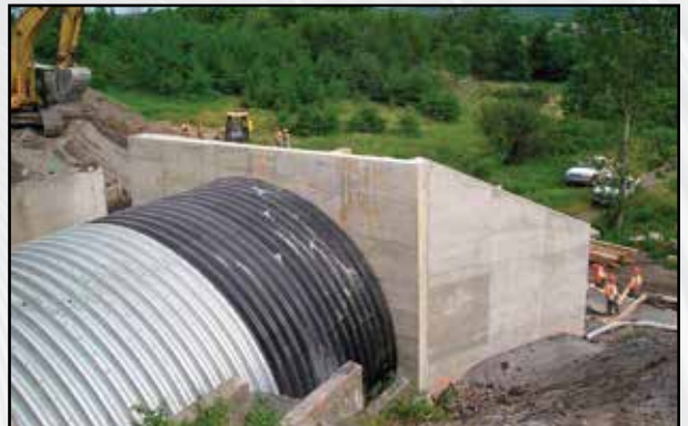
Vehicular Underpass with Top Plates Polymer Coated for Deicing Salt Runoff from Major Highway
