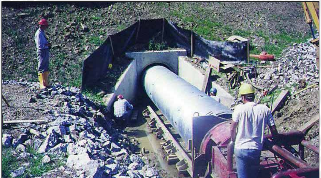
JACKING CORRUGATED STEEL PIPE INTO CONCRETE PIPE HIGH FILL REPAIR SITUATION
