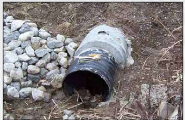
POLYMER LAMINATED CSP RELINE PIPE FULLY GROUTED
