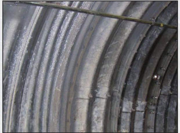
TUNNEL LINER PLATE WELDED TO CSP
