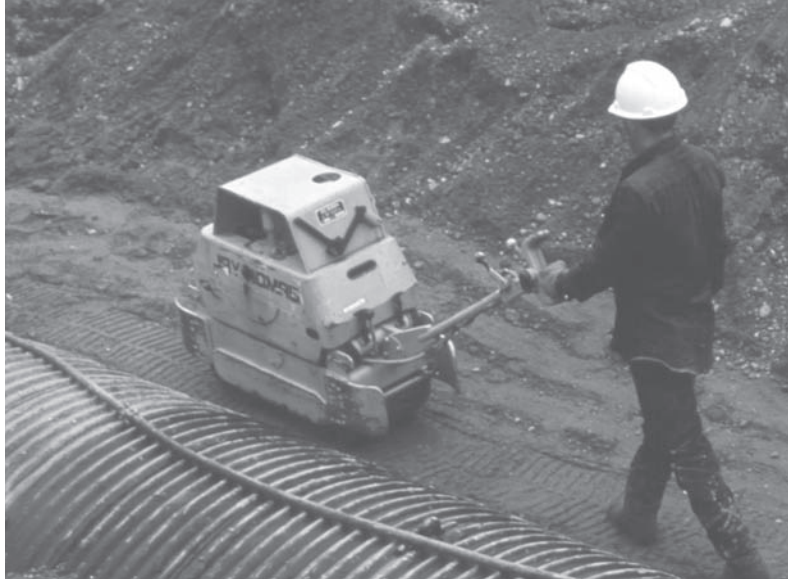
Adequate, uniform compaction is the secret to building soil and steel structures.
