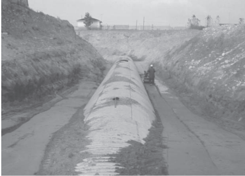
Trenches should be wide enough to permit proper tamping of backfill.
