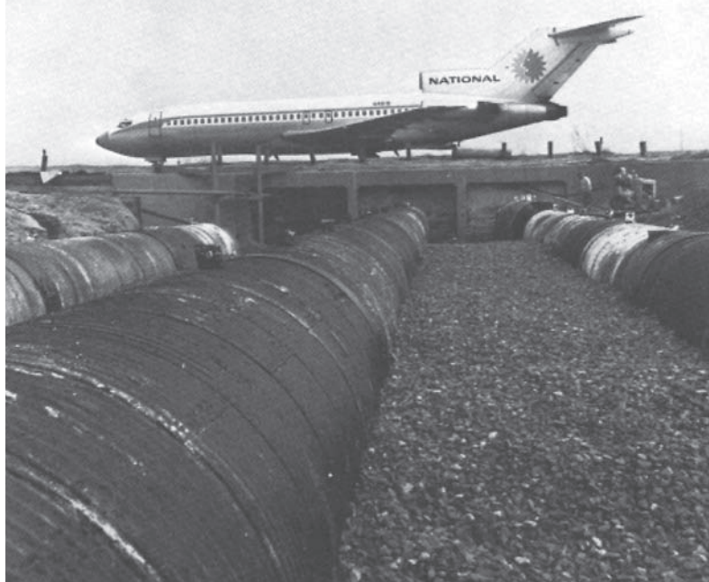
CSP was a cost effective solution for the Newark Airport.
