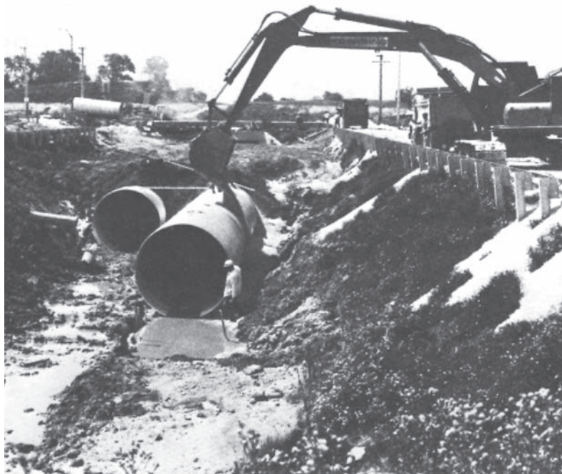
Plain galvanized CSP satisfied service life requirements for storm drains in this environment.
