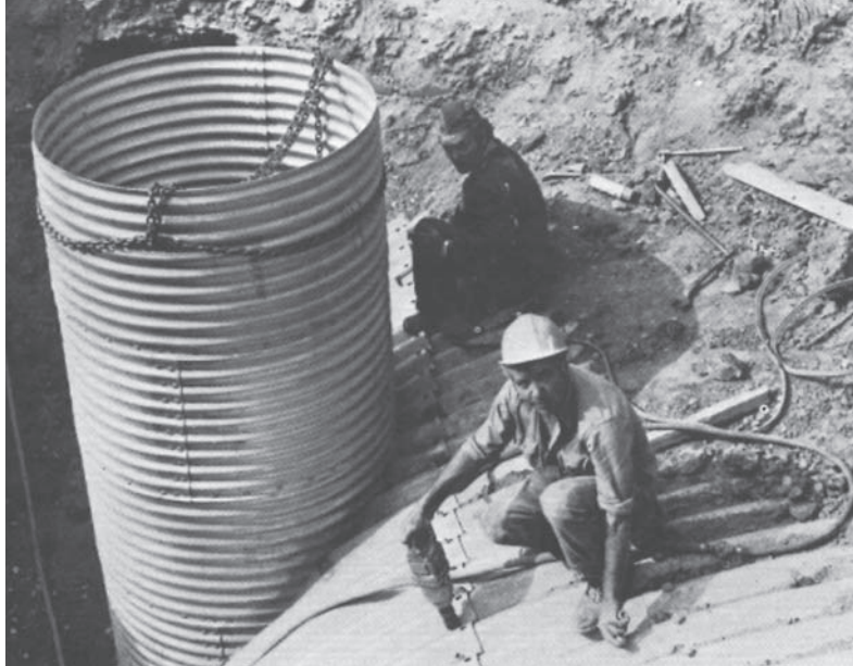
Joining factory made CSP to large structural plate storm drain.
