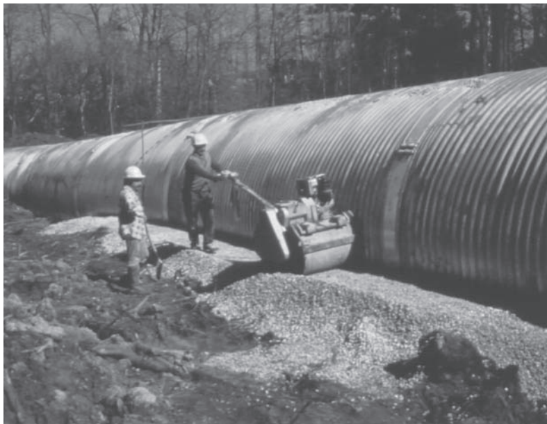
Compacting backfill is required for proper installation of all sewers.
