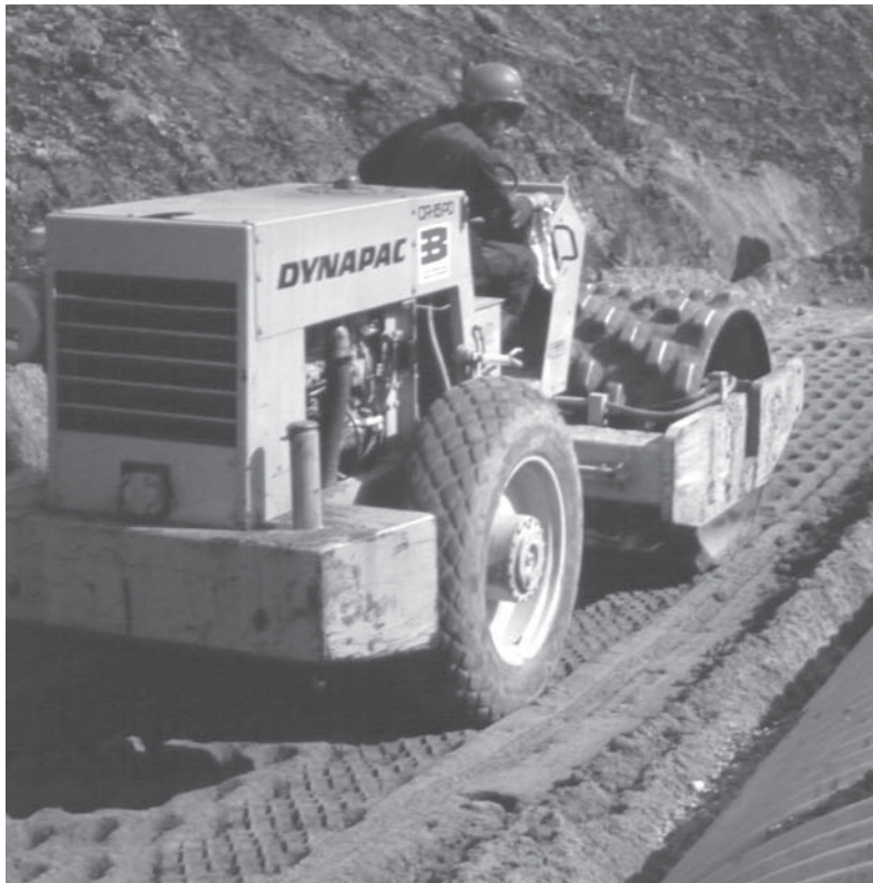
Proper installation techniques are always important.
