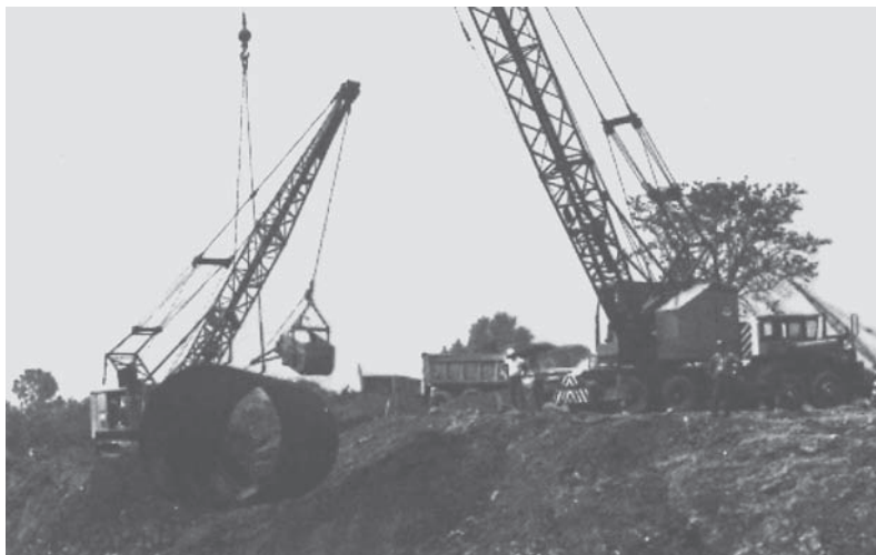
CSP is easy to install in difficult trench conditions.
