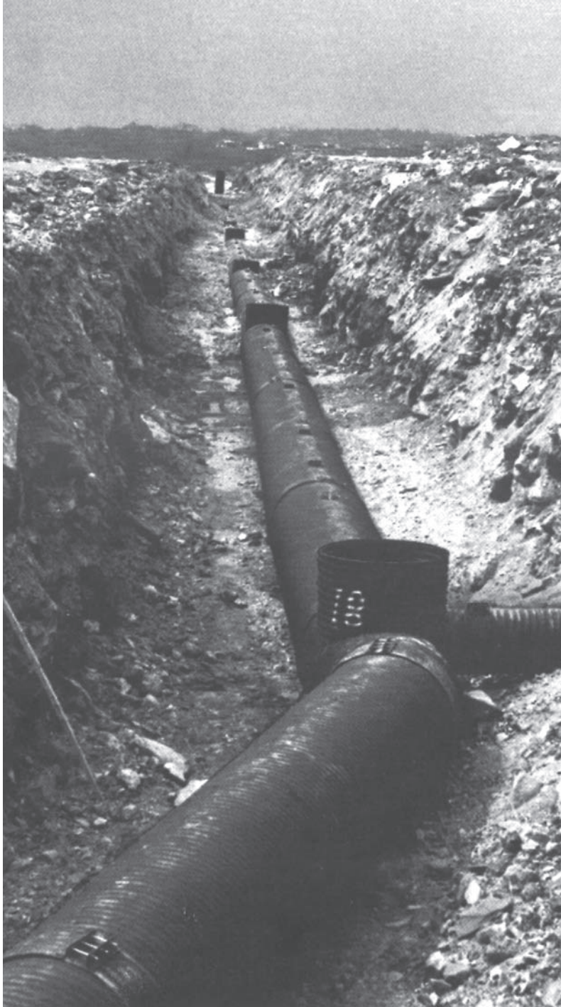
Fabricated fittings reduce head losses in the system.
