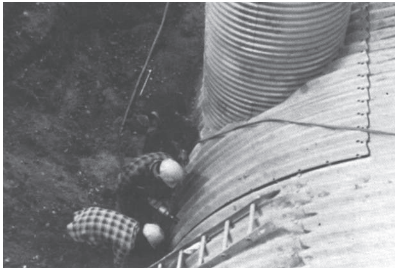
Saddle branch manhole is bolted in place.
