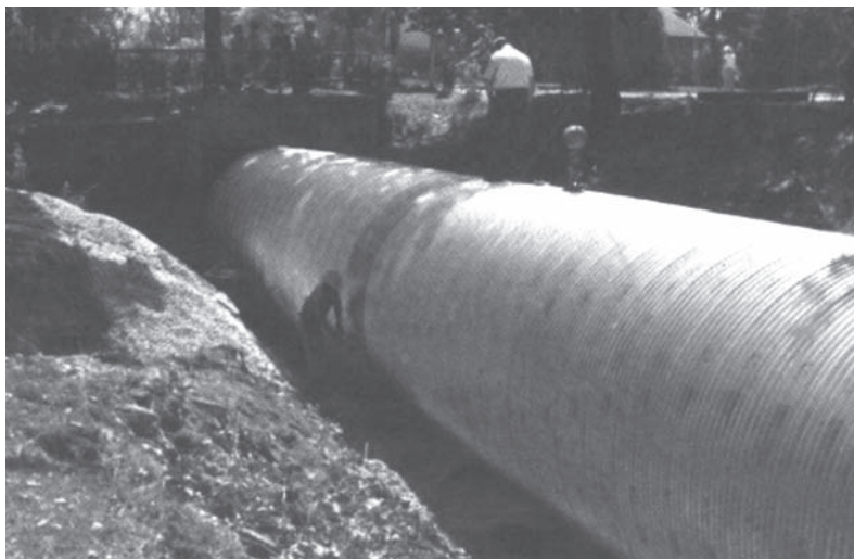
Ease of installation of CSP through existing concrete box.
