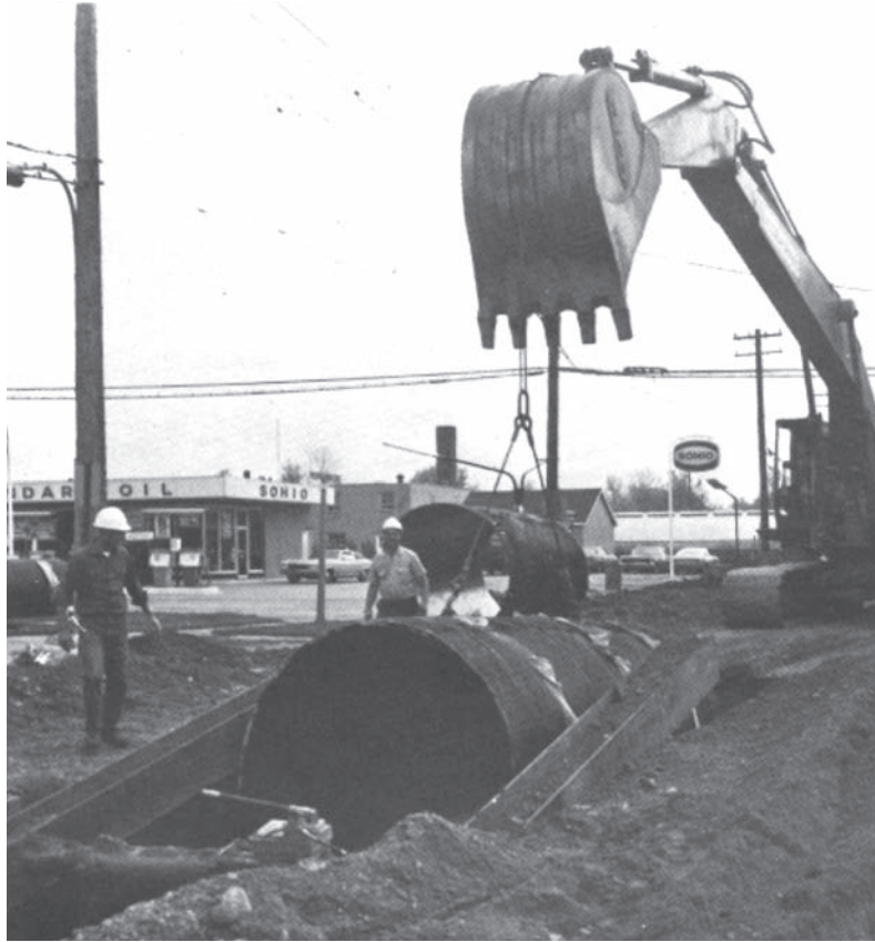
Laying Full Bituminous coated and Full Paved CSP.
