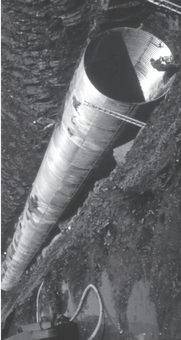
7 m diameter steel sewer being installed in wet conditions.
