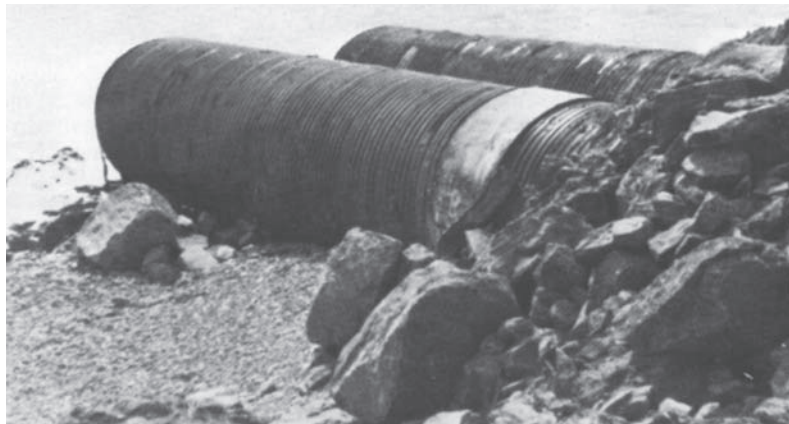
Twin outfall lines for major urban storm sewer system.
