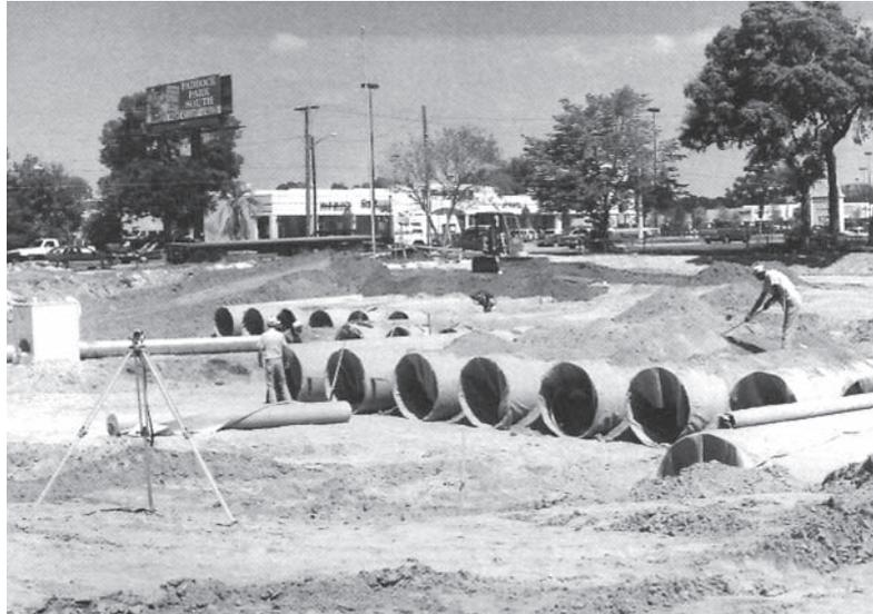
*A view of the 18 lines of 1200 mm diameter fully perforated corrugated steel pipe used as a recharge system.*
