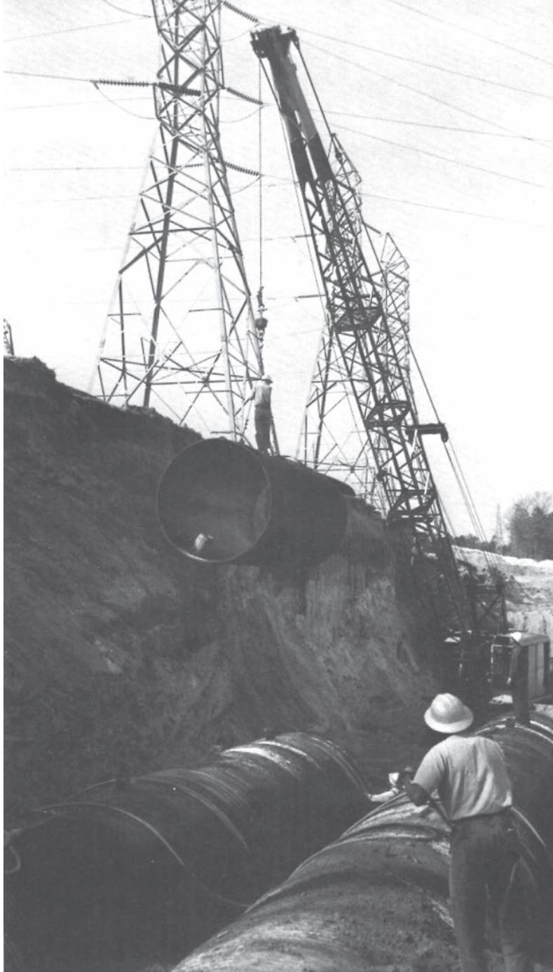
*Twin 180 m long smooth line, 2400 mm diameter provide cooling water at the Crist Steam Generating Plant of Gulf Power Company.*
