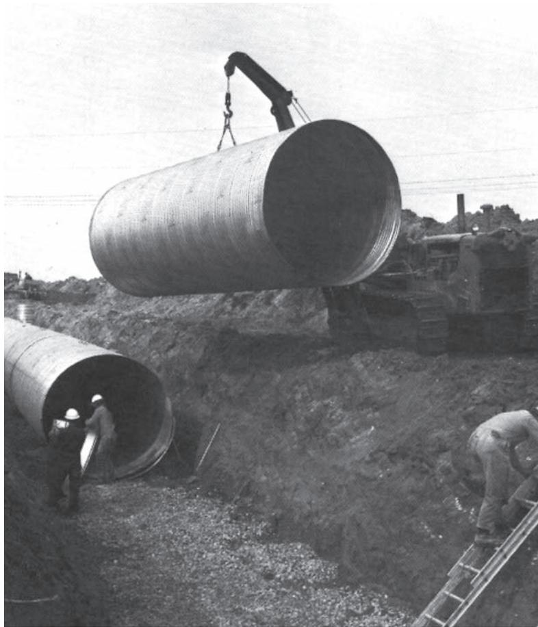
*Long lengths with fewer joints can lower the effective "n" value.*
