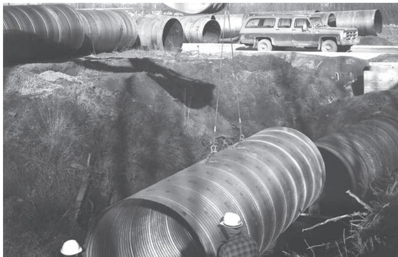
*Lifting lugs are provided to protect the exterior coating on this CSP.*
