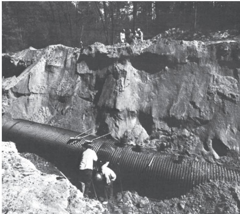
*Standard CSP structural designs permit unrestricted trench width.*
