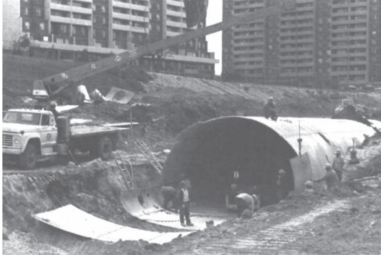
Structural plate storm sewer encloses stream in an urban area.
