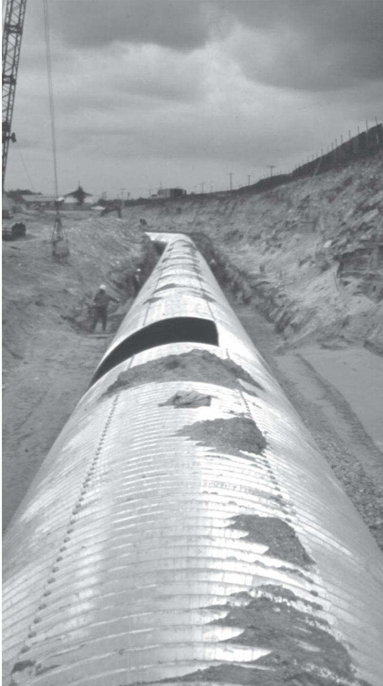
*CSP Sewer designed for very wide trenches.*
