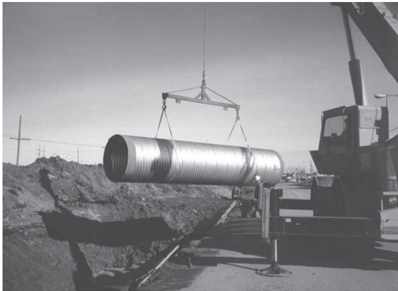
*Exterior coatings are protected during installation by use of lifting lungs or slings.*
