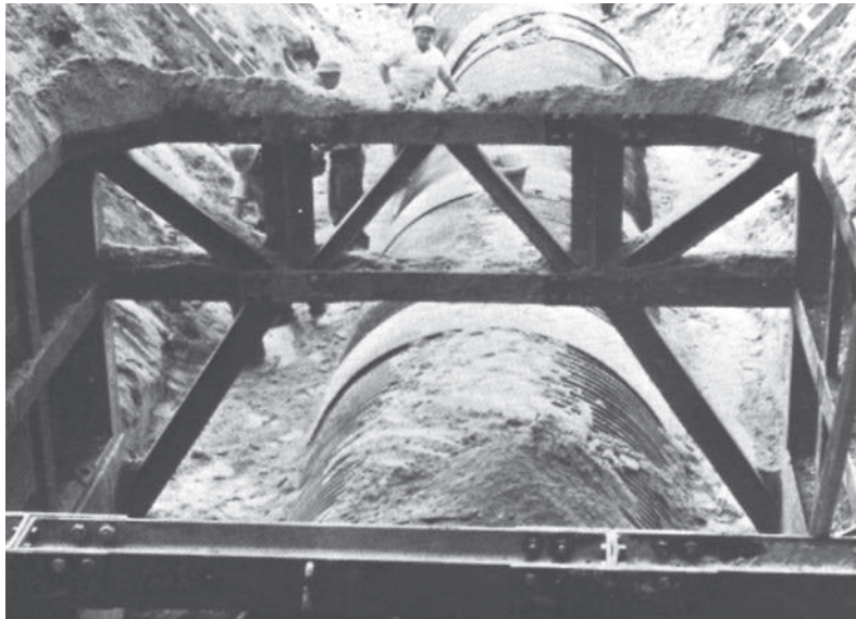
Using steel trench shield to install CSP sewer.
