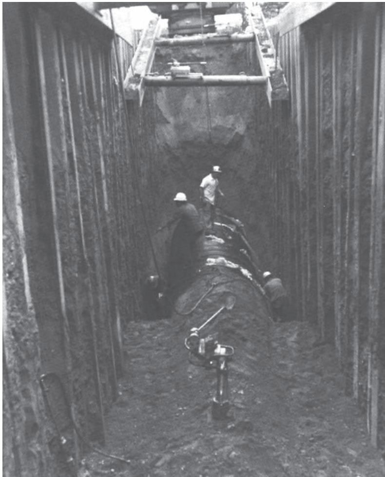
76mm x 25mm full bituminous coated and full paved storm sewer, 820m, 2200mm diameter, 1.6mm.
