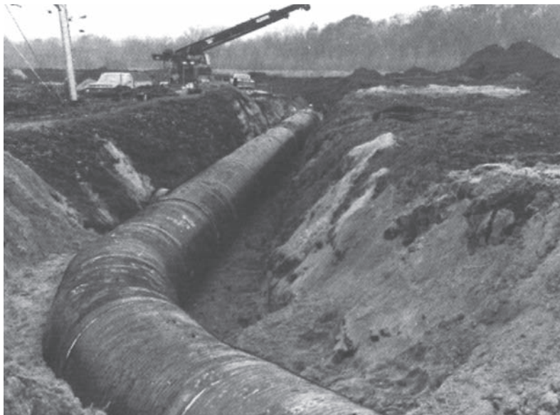
Installation of CSP sanitary sewers.
