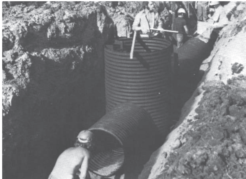
Manhole risers can be built into the sewers with CSP pipe.
