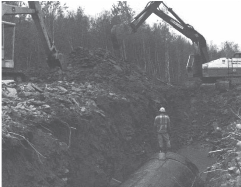
Quick installation of CSP sewer keeps pace with modern trenching equipment.
