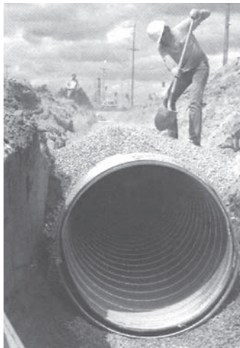
Spiral rib pipe installation.
