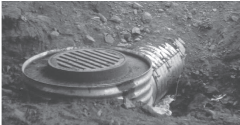
Standard cast iron covers and/or steel grates are used with CSP manholes and catch basins.
