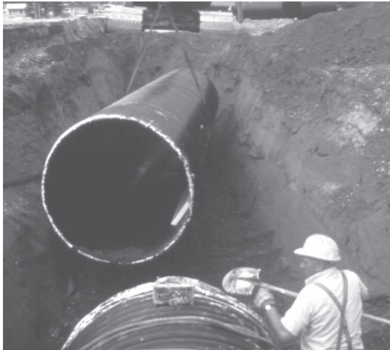
Placing coated CSP sewer section. Fabric sling protects pipe coating.
