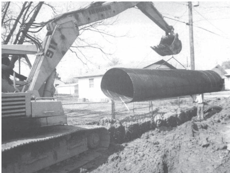
Lengths of pipe arch are easily moved into position.
