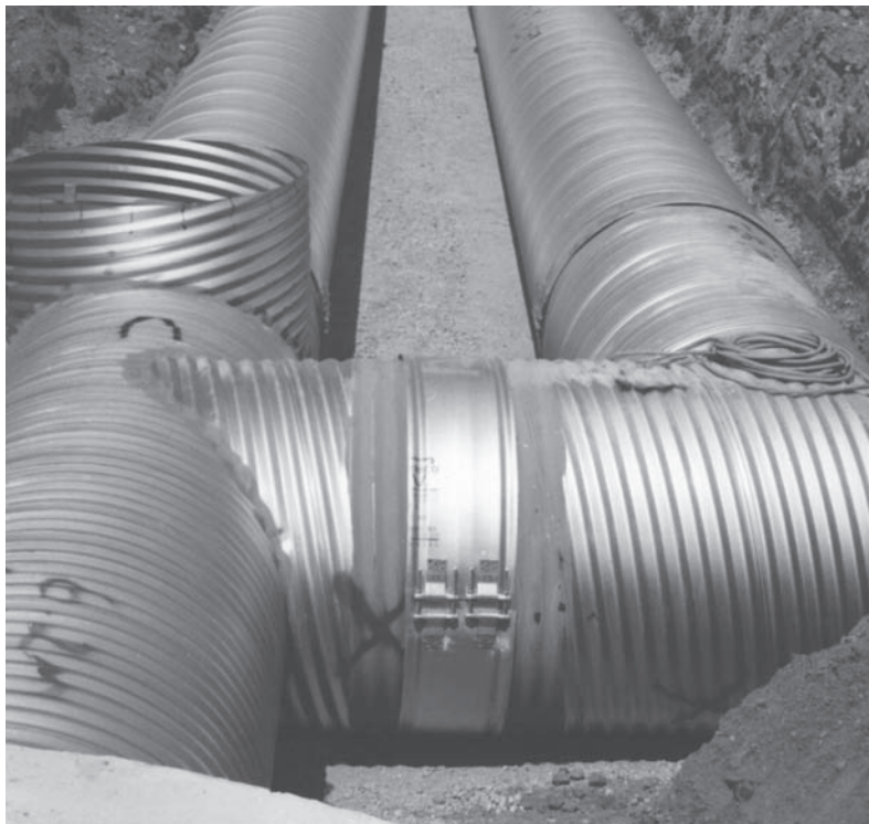
Common manifold eliminates costly junction box used with other storm drain materials.
