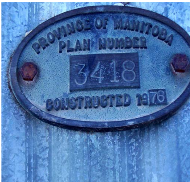
Date Plaque on Highway Culvert
