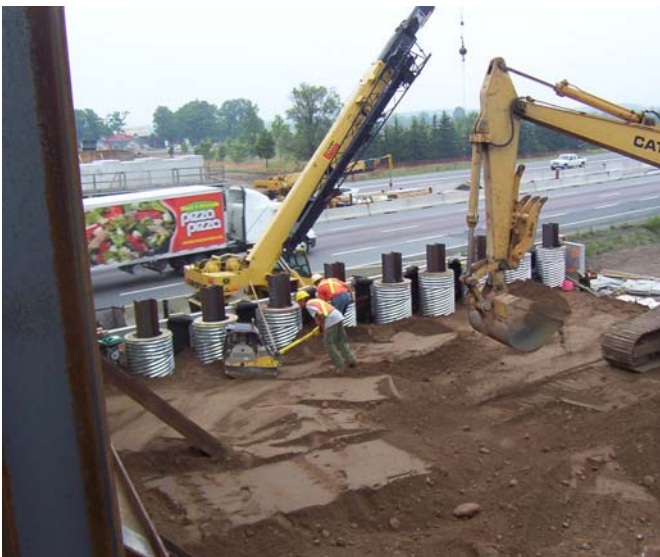
Compacting Fill Against the Caissons
