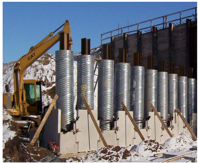
Second Phase of Overpass Replacement
