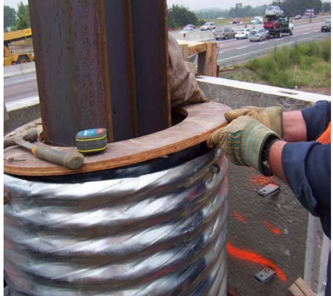
Closing in the Caisson
