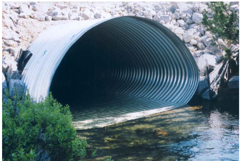
Corrugated Steel Pipe Arch 3650mm x 2280mm, 3.5mm Aluminized Type 2 Steel
