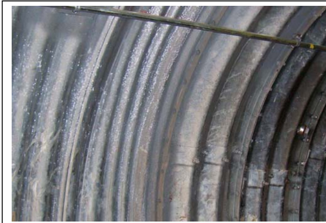
Tunnel Liner Plate Welded to CSP
