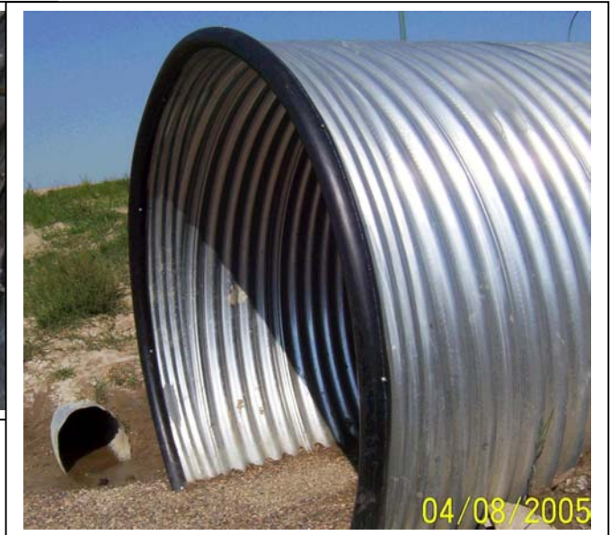
Tunnel Liner Plate Welded to CSP
