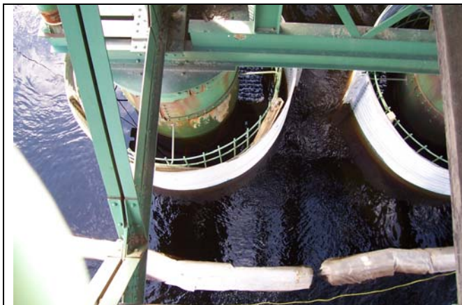
Caissons & Reinforcing Steel in Place
